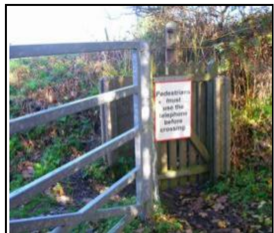
Figure 12: View of wicket gate with sign advising pedestrians to use the telephone before crossing. November 2013
