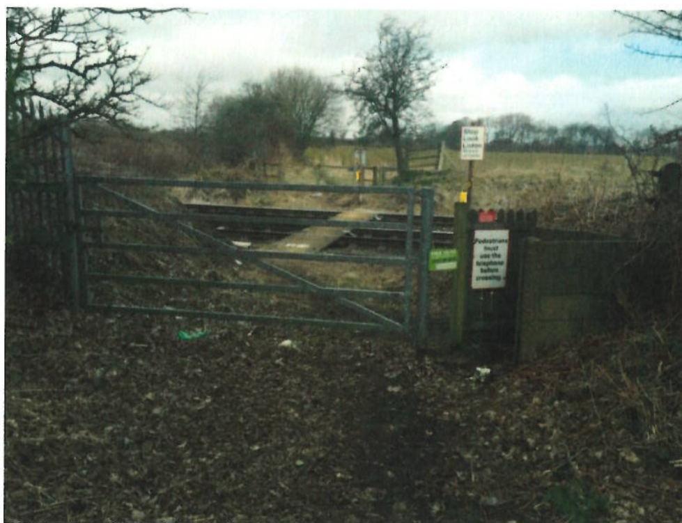
Fence / gate to south of crossing
