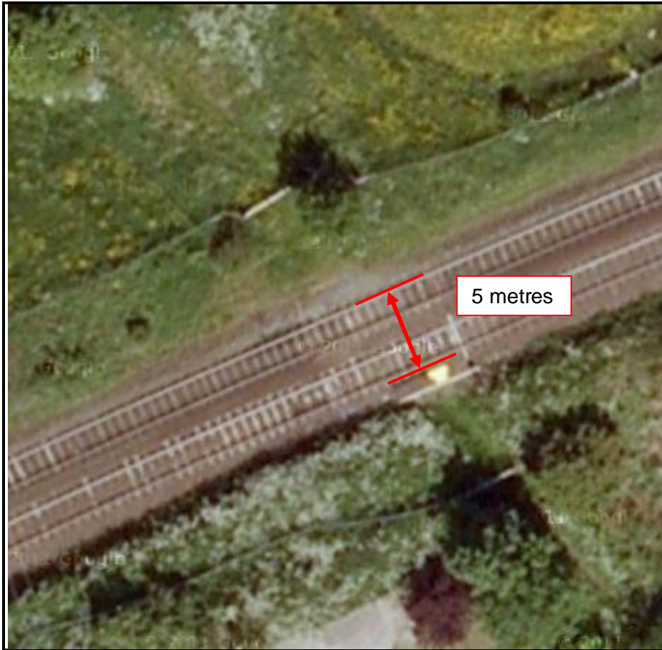
Figure 28: Aerial image of Moss Lane Farm level crossing with dimension. Image taken from Google footage.
