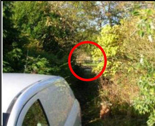
Figure 9: Moss Lane travelling towards Moss Lane Farm level crossing. The red circle highlights the gate at the crossing. The vehicle on the bottom left corner is the closest position a vehicle could get to the crossing. November 2013
