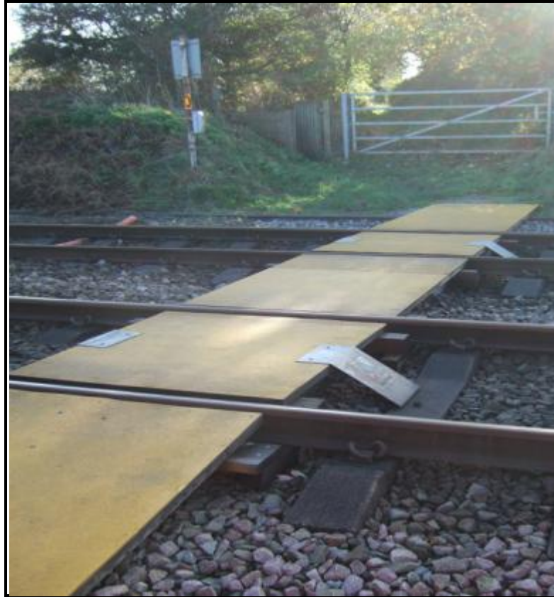
Figure 3: Moss Lane Farm level crossing looking south, November 2013
