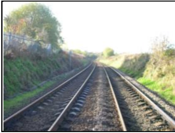
Figure 22: Down to Ashton Under Lyne approaching the crossing on the right side of the image. View from centre of Moss Lane Farm level crossing looking west. November 2013
