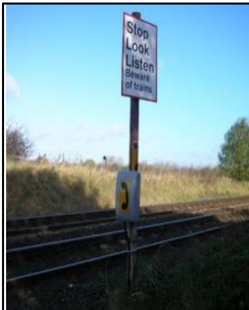
Figure 19: Stop Look Listen sign and telephone located on the south side of Moss Lane Farm level crossing. November 2013
