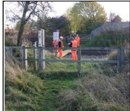
Figure 16: View of footpath approaching a fixed fence in the centre of the image and wicket gate on the left side of the image. November 2013
