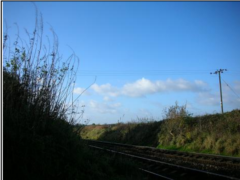
Figure 27: Image of overhead lines passing over the railway, taken from Moss Lane Farm crossing looking west. November 2013
