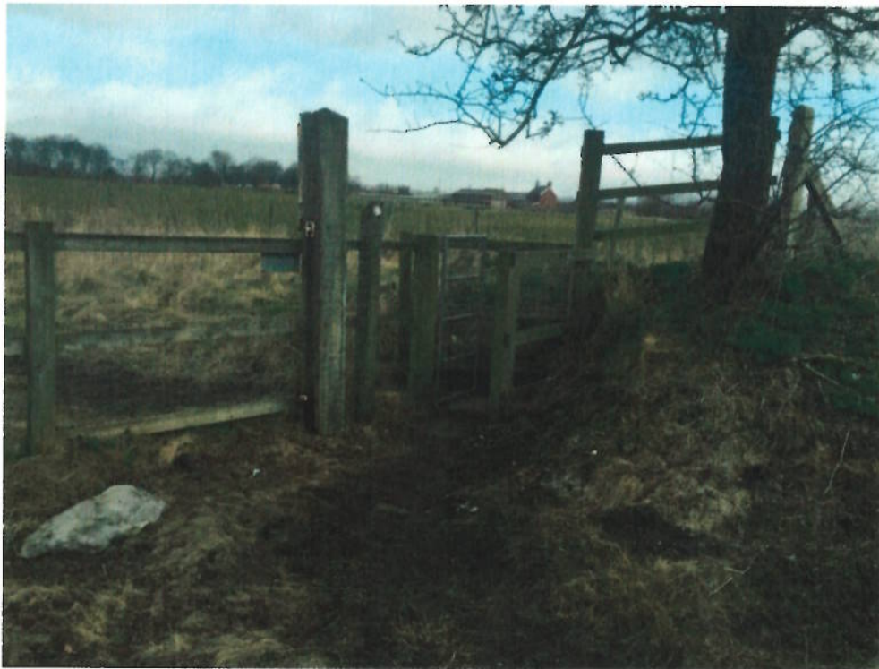
Fence / gate to north of crossing
